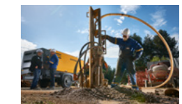
14 bar: blast hole drilling or ground engineering drilling
